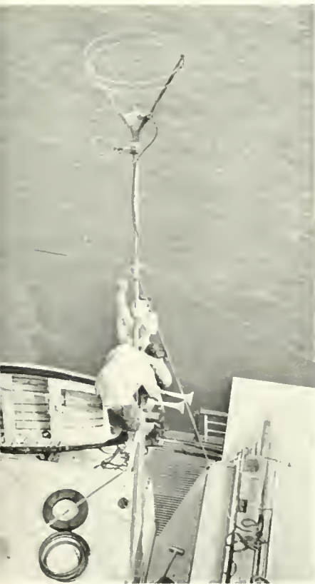
RCA TECHNICIANS ERECTING THE TELEVISION ANTENNA ABOARD THE PILOT BOAT NEW JERSEY. THE SMALL LOOP BELOW THE LARGE ANTENNA IS FOR STATIONS ON CHANNELS 7 TO 13.
